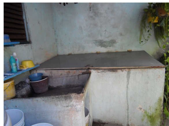
Fig. 3 A covered concrete water storage tank ( pila )
