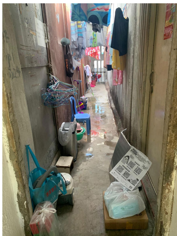
Fig. 1 Corridor of SDUs with shared laundry space
