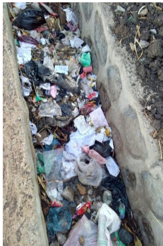
Fig. 2 Waste disposed of in Ditches (Around Welkesa Kebele) of Asella town, 2017. (Image taken by the corresponding author)
